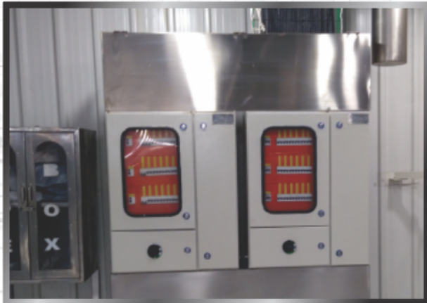
POWER DISTRIBUTION BOARD WORK
