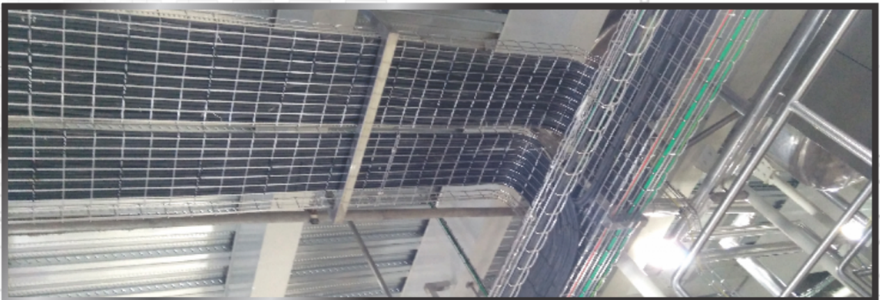
CABLE TRAY WORK
